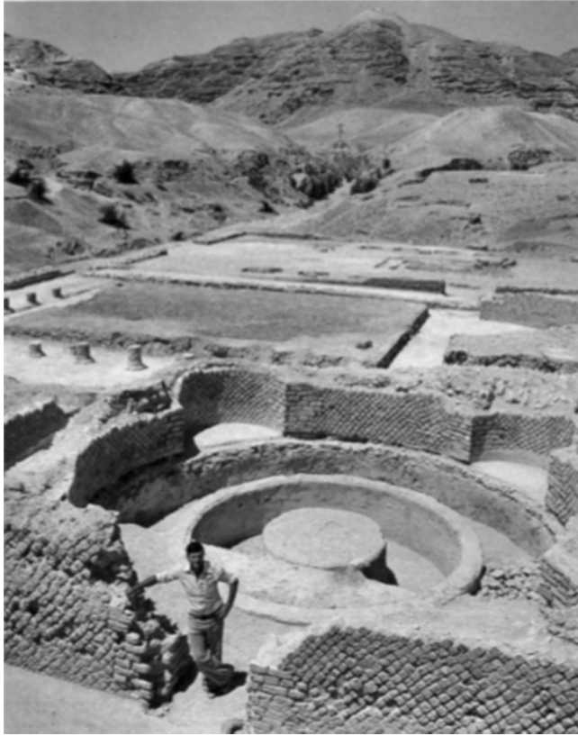
Fig. 4. Photograph of the Ehud Netzer standing at the entrance of the laconicum of the bathing suite in Herod's Third Palace at Jericho. The walls are faced with opus reticulatum and opus quadratum .
