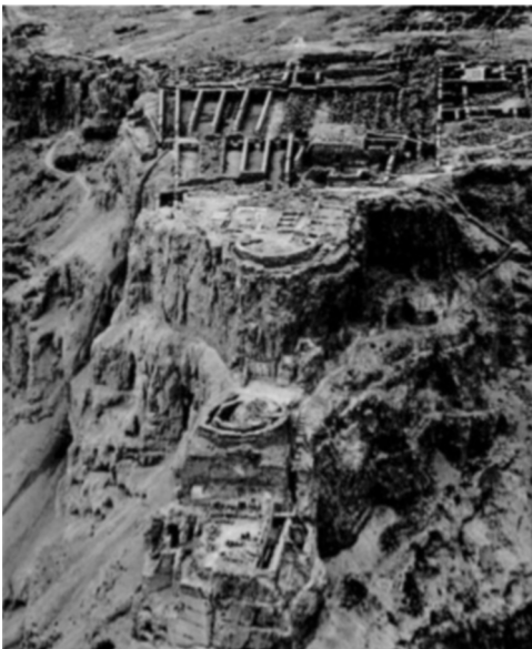
Fig. 6a. View of the Northern Palace of Masada from the north, showing the remains of its constituent sections, built on three levels.
